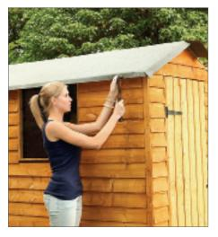
E Add the roof beam across the top of the shed, fitting it to the pre-cut grooves on each gable end. Check that the shed feels firm to the base and that the door opens easily. Find the L shaped bracket and use 30mm screws to fix the beam to each gable end.
